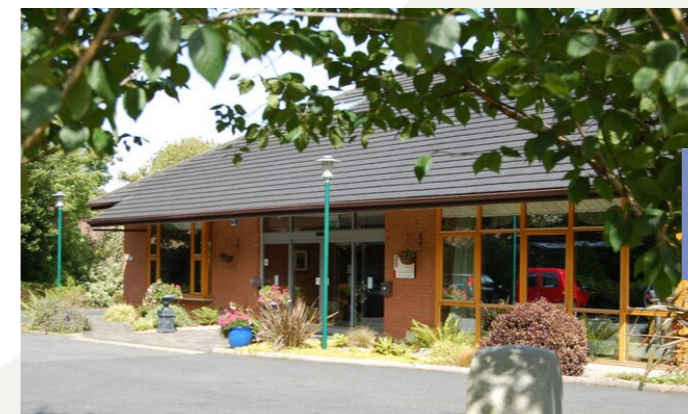
Cheshire Ireland social housing units in Waterford city
